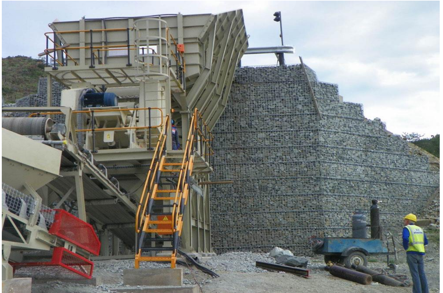
Queenstown Quarry : New crusher installation R30 million
