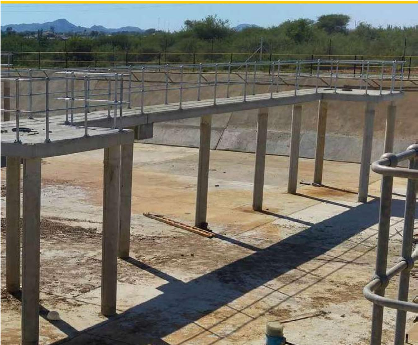
Deepening of the stormwater holding tank by another metre (February 2016).
